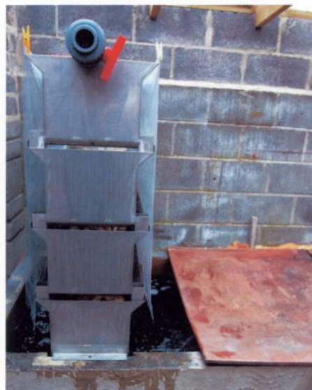
Dave's older generation Bakki Shower currently sits over the pump bay, but will soon be moved so that the water returns directly to the pond. The polythene is to avoid the water splashing, which was a minor drawback with this older 'Mark II' version. Beneath the Shower you can see the three pipes that take the water back to the pond, returning close to the floor at the shallow end
